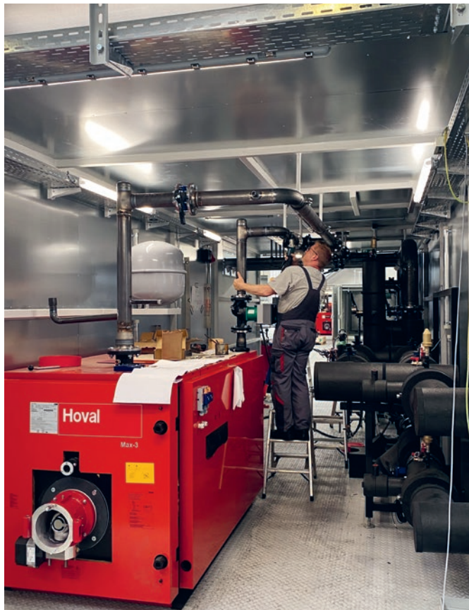
Assembling an energy centre.
