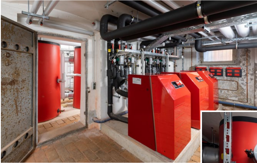
The new heating centre consists of an UltraGas® gas condensing boiler, three Thermalia® heat pumps and one combined heat and power plant (CHP plant).
