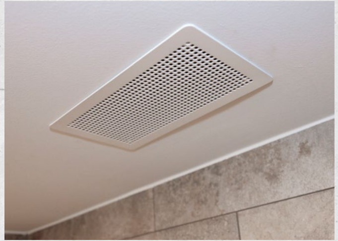
Each of the newly renovated flats is fitted with an autonomous HomeVent® comfort ventilation unit.
