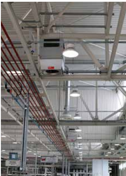
Decentralised recirculation units without ventilation ducts can be integrated into the infrastructure of large spaces without becoming a hindrance to other systems (shelving, crane runways, lighting, and so on).
