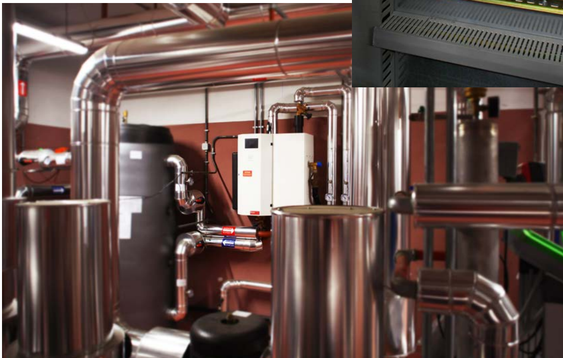
The system controller components are located in a control panel. The TransTherm® aqua F provides hot water in the seminary.
